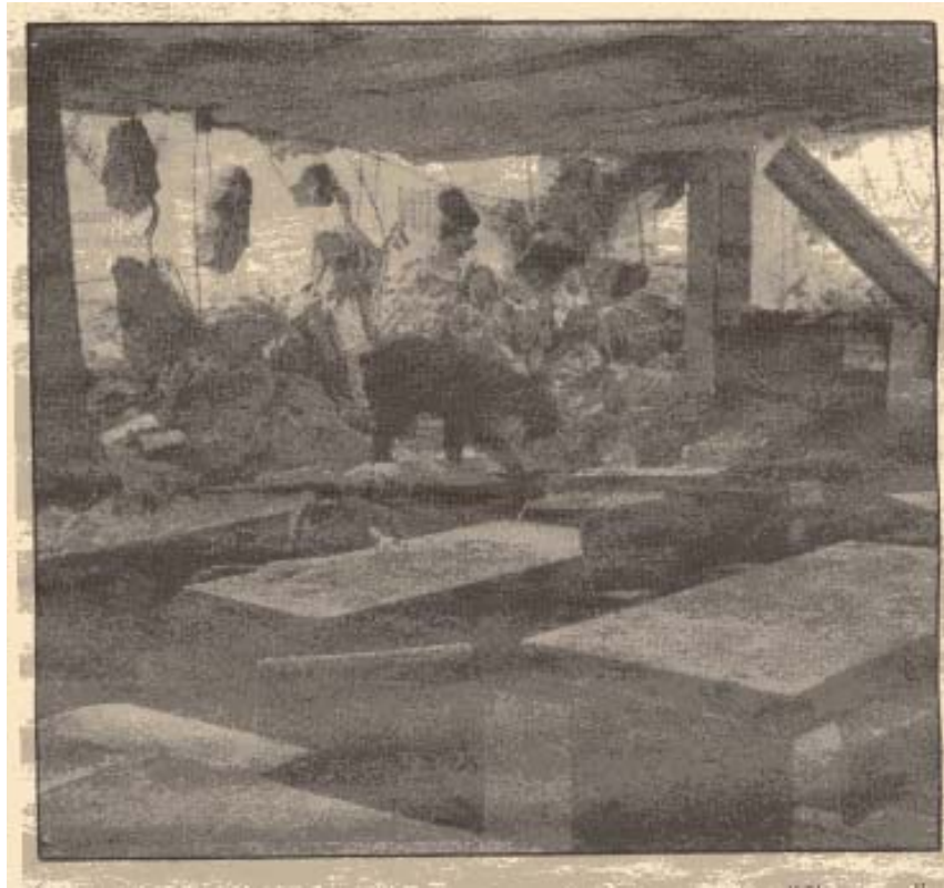
Berry searches an office building. Half the structure had collapsed. Betty Blake photos.
